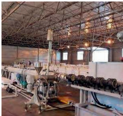
Production line of sewer and delivery pipes with a diameter of 16, 20, 25, 32, 40, 50, 63 and 75 mm. Productivity of this line is 800-1000 kg per day.
